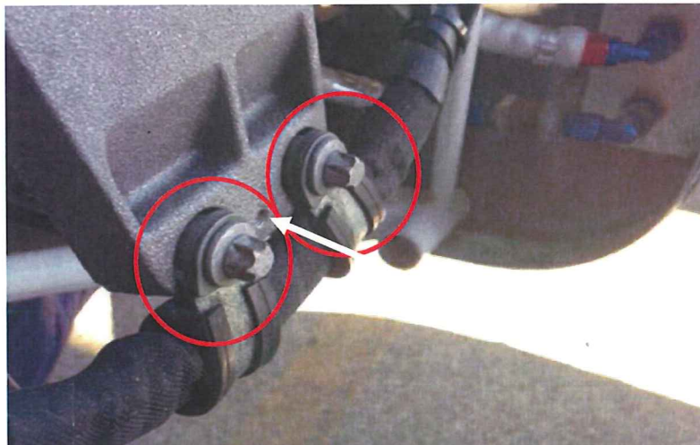
Figure 1: WRONG mounted alternator loom
